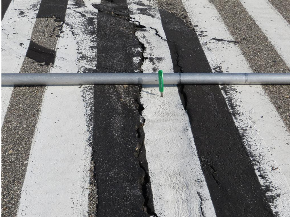
Y63 RY1432 001 (L&T Crack > 3 inches filled with sealant)
