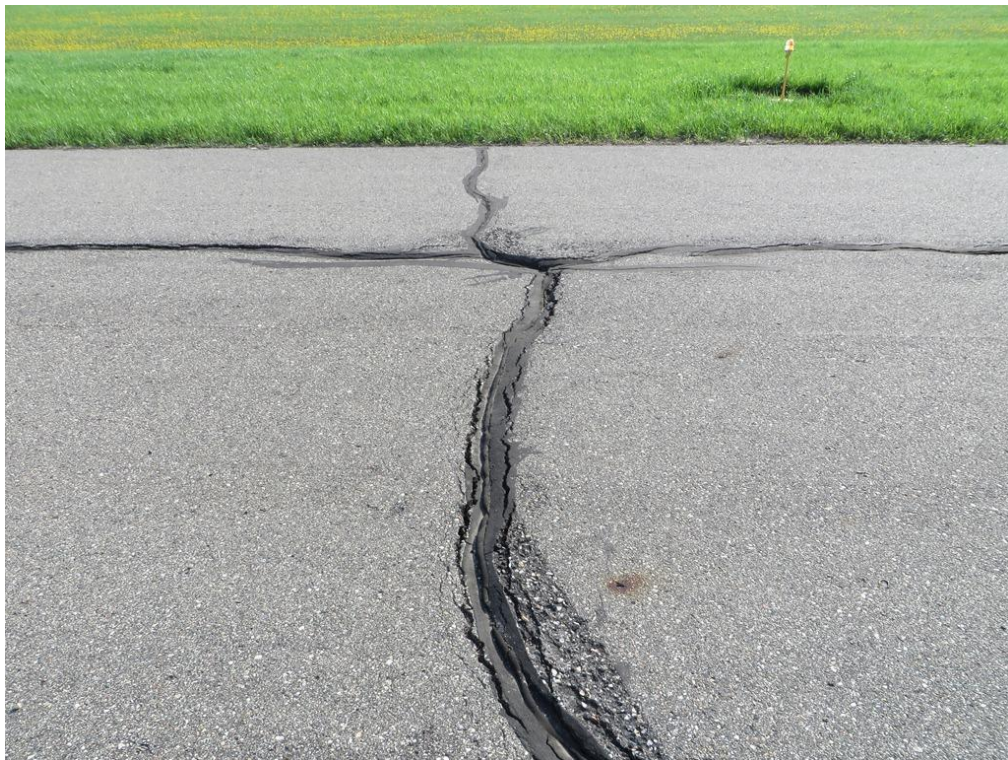
Y63 RY1432 001 (L&T Cracking with Subsidence)
